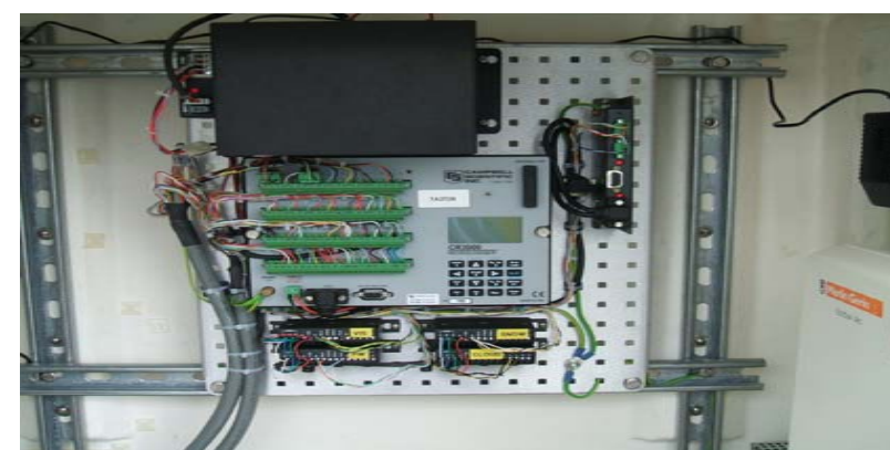
Inside the workings of an MMS site with the CR3000 logger and the feeds from the various sensors into it.
