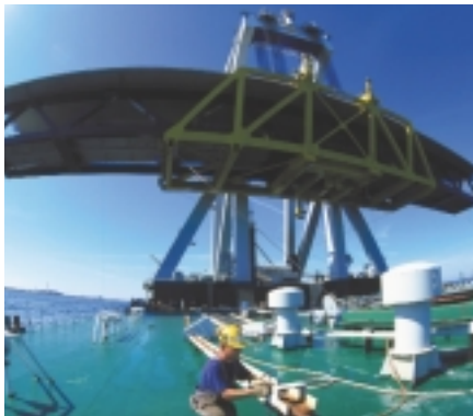
Construction of the Øresund Bridge.
